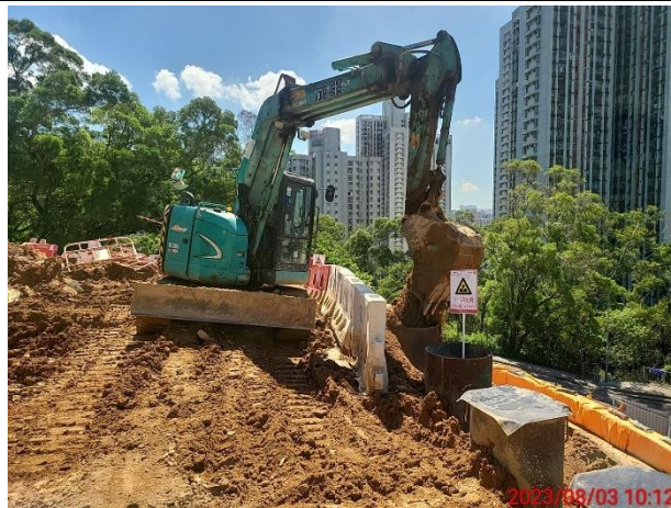
Construction activities: Backfill
