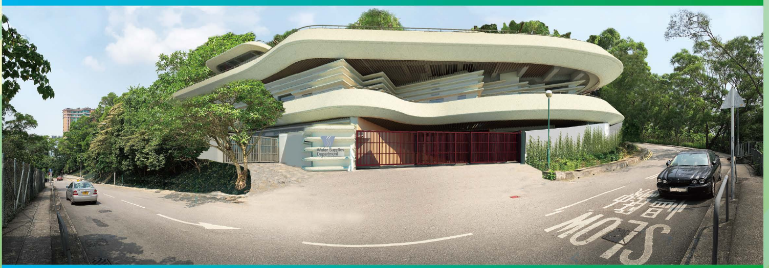
擬建於連接隧道入口的通風設備及其他相關機電設施 Proposed Ventilation and Other Associated E&M Facilities at Access Tunnel Portal Area
